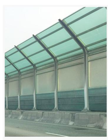
Reference Image: Noise Barrier at Fanling Highway with curved steel frame
